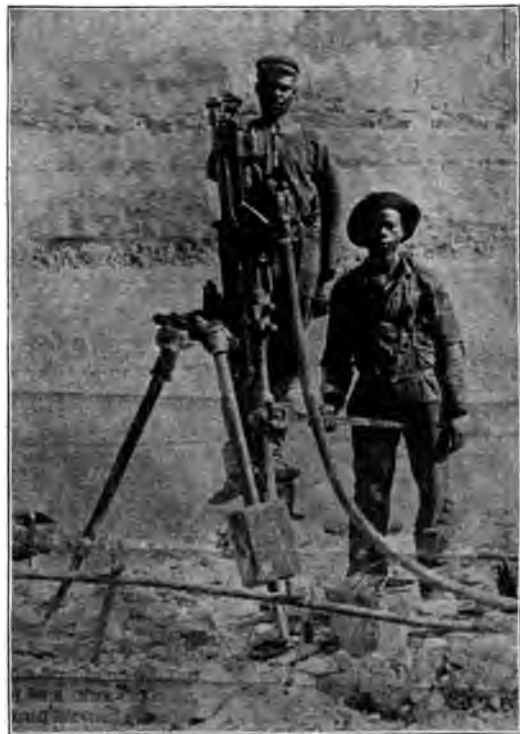
COMPRESSED-AIR DRILL, CHICAGO DRAINAGE CANAL.
